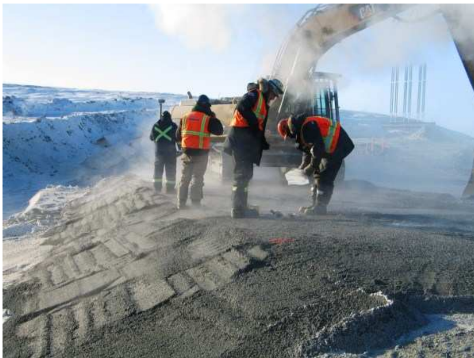
Photo 7: Initial placement of core material on slopes. Station 0+100 facing south
