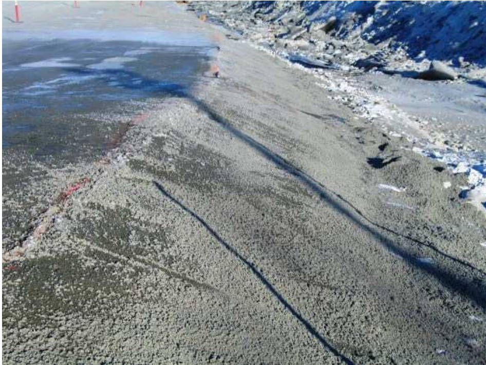
Photo 8: Hand raked backslope Sta 0+73 facing north
