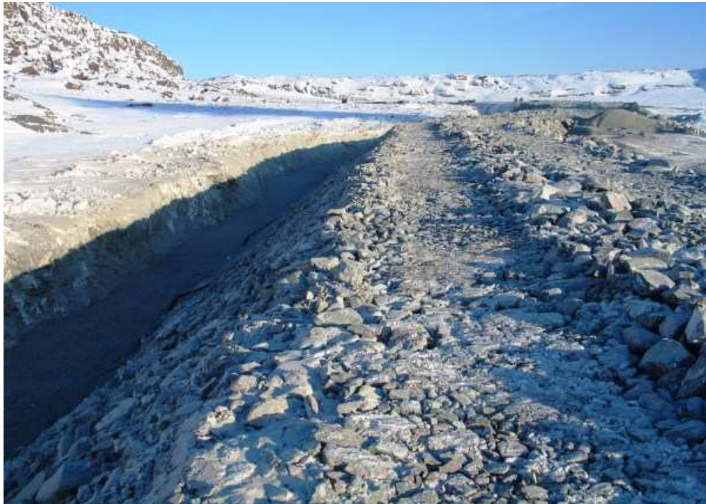
Photo 12: Crush levelling course ~ Sta 0+300
