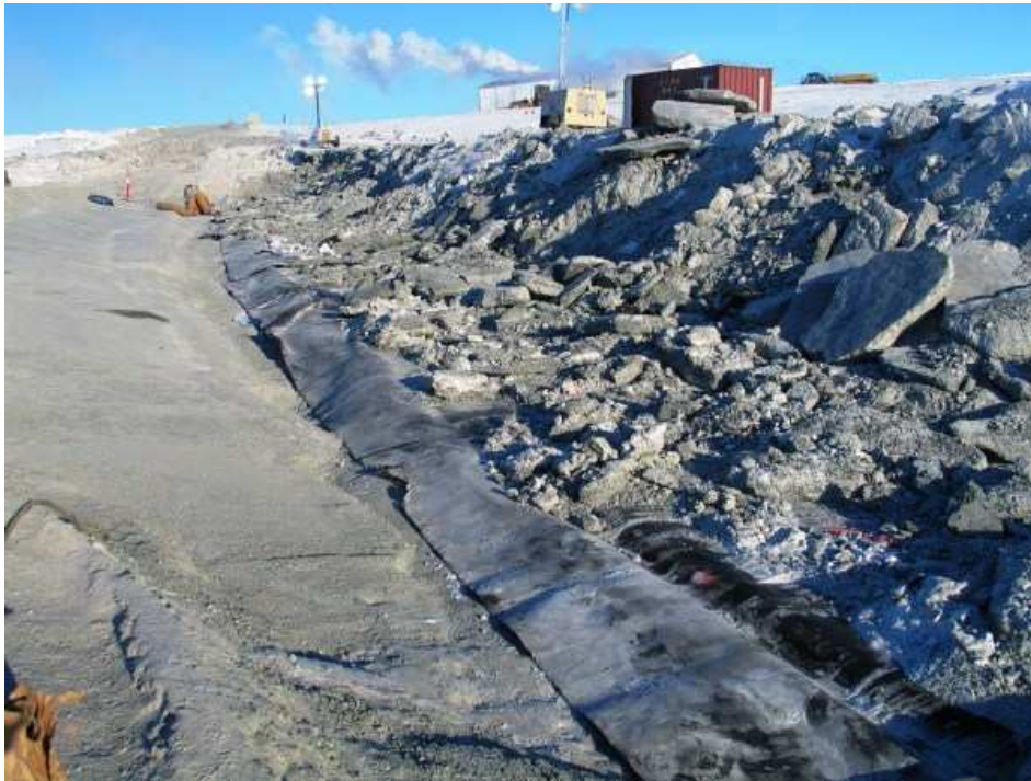
Photo 10: ROQ removal over HDPE Station 1+30 facing north
