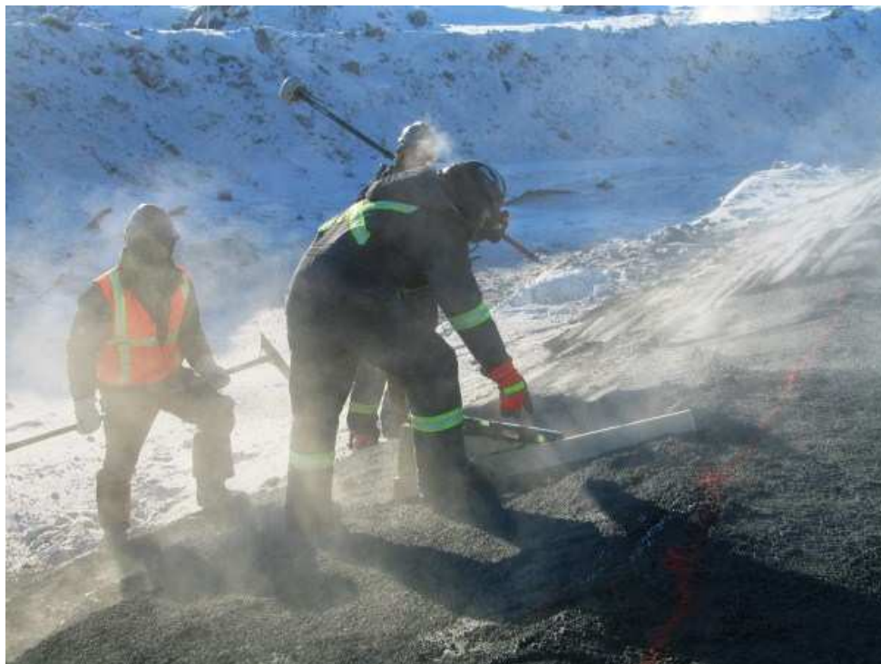
Photo 9: Hand raking. Note device being used to establish angle
