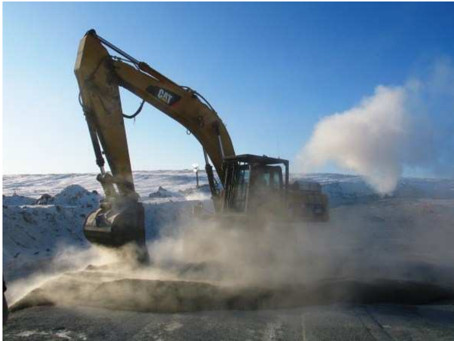
Photos 6: Placing frozen core material at Station 0+100
