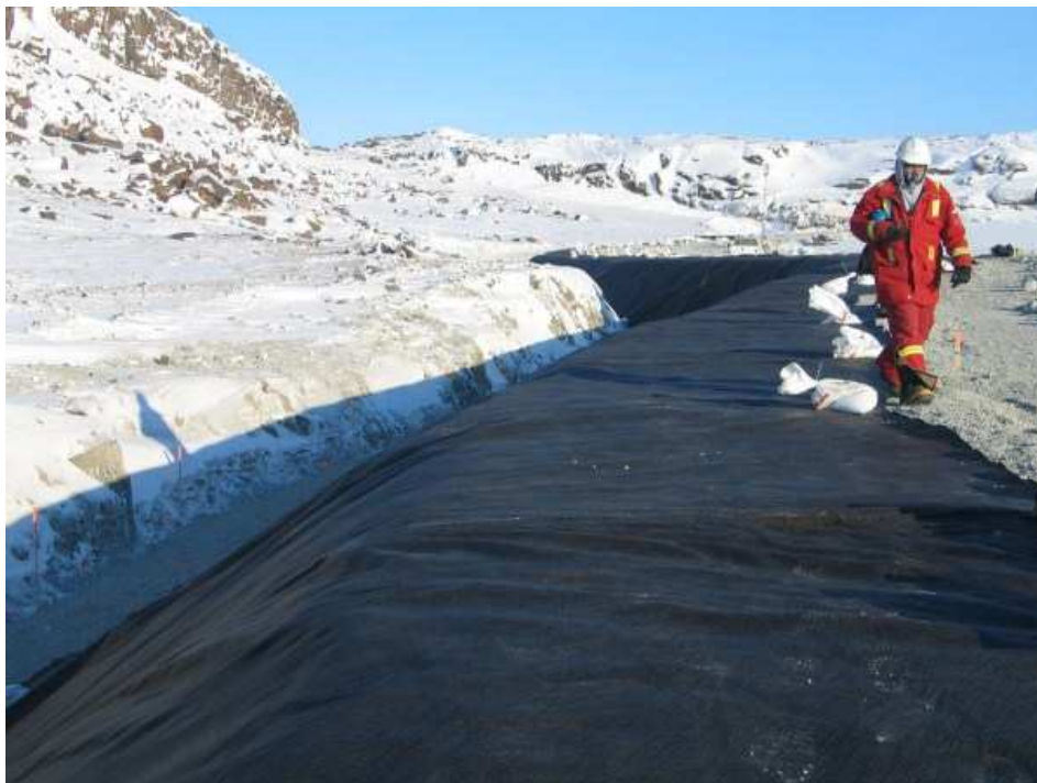
Photo 11: Geotextile placed to Sta 0+445 facing east,
